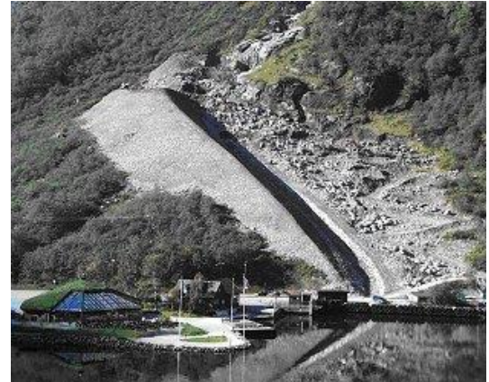
avalanche deflecting dams in western Norway (photos: NGI)
